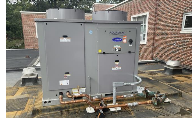
Hampton Roads AREC Chiller Replacement
