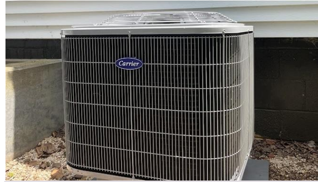
Middleburg AREC Employee House 816 Heat Pump Replacement
