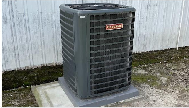
Tidewater AREC Entomology Lab Heat Pump Replacement
