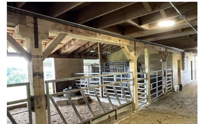
Beef Barn Structural Repairs
