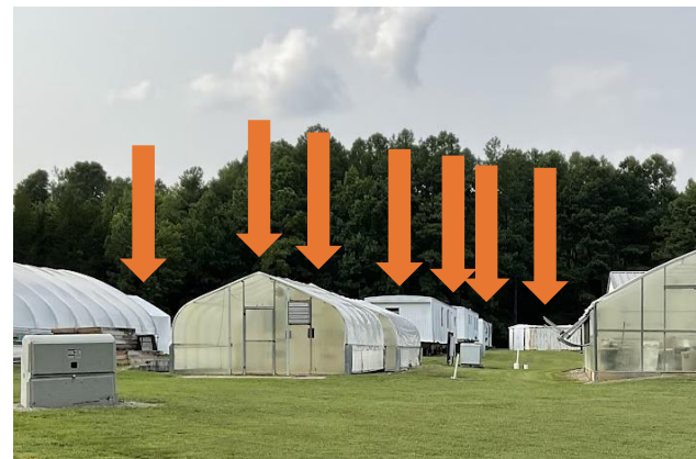
SPAREC Building removal
