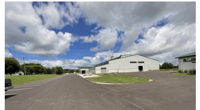
Alphin-Stuart Livestock Arena Parking Lot Paving
