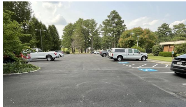
Southern Piedmont AREC Road and Parking lot Repaving
